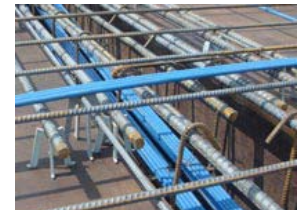
Slab tendon passing over bundled tendons in a P-T beam
