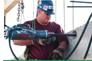
Tendon being "jacked" to induce tension
