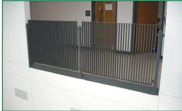
handrail assembly, one may find the handrail to be 'wobbly'. Even though the deflection at the top of the edge angle is very small, the deflection at the handrail, a few feet above, may not be.
