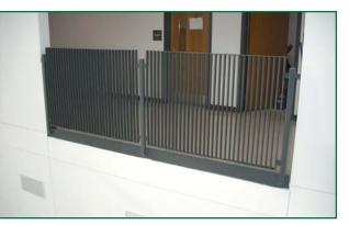
handrail assembly, one may find the handrail to be 'wobbly'. Even though the deflection at the top of the edge angle is very small, the deflection at the handrail, a few feet above, may not be.
